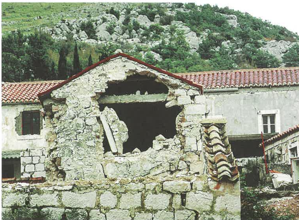
Slika 5. Obsežne poškodbe starejše hiše v vasi Podimoč. Porušil se je nosilni zid. Fig. 5. Extensive damage to an older house in the village of Podimoč. The main pillar wall was destroyed.
