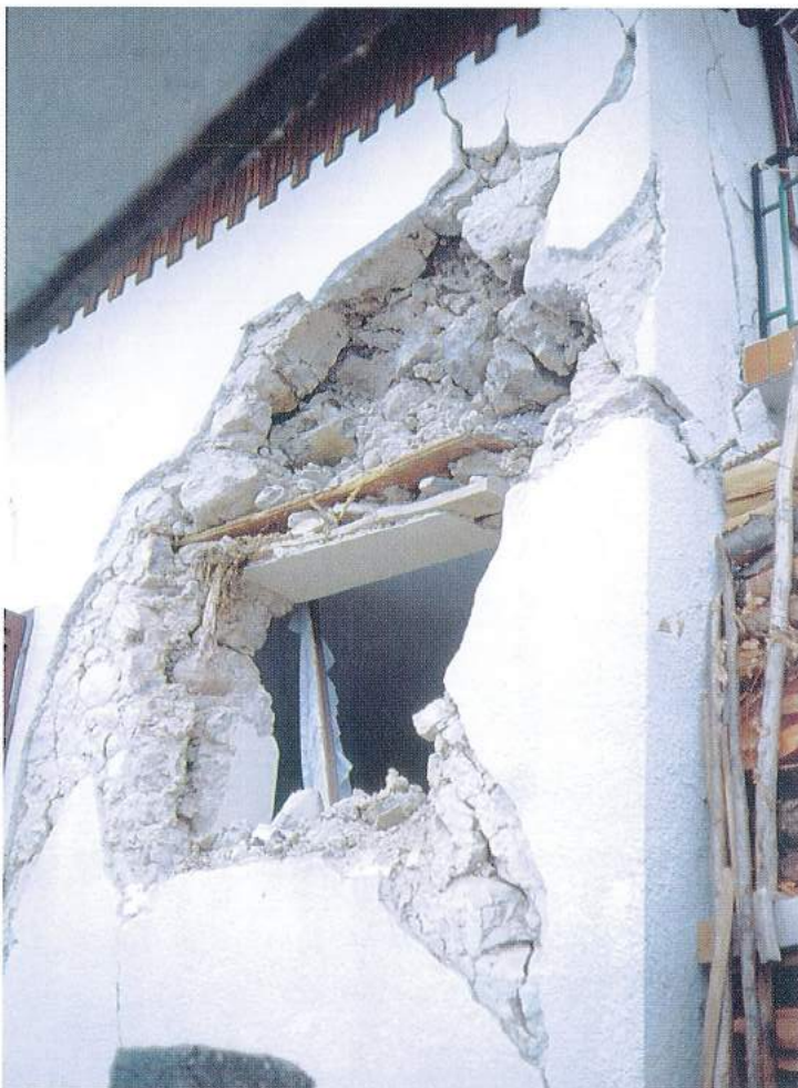
Figure 12. Completely destroyed building on the Polog mountain above Tolmin (damage of grade 5).
