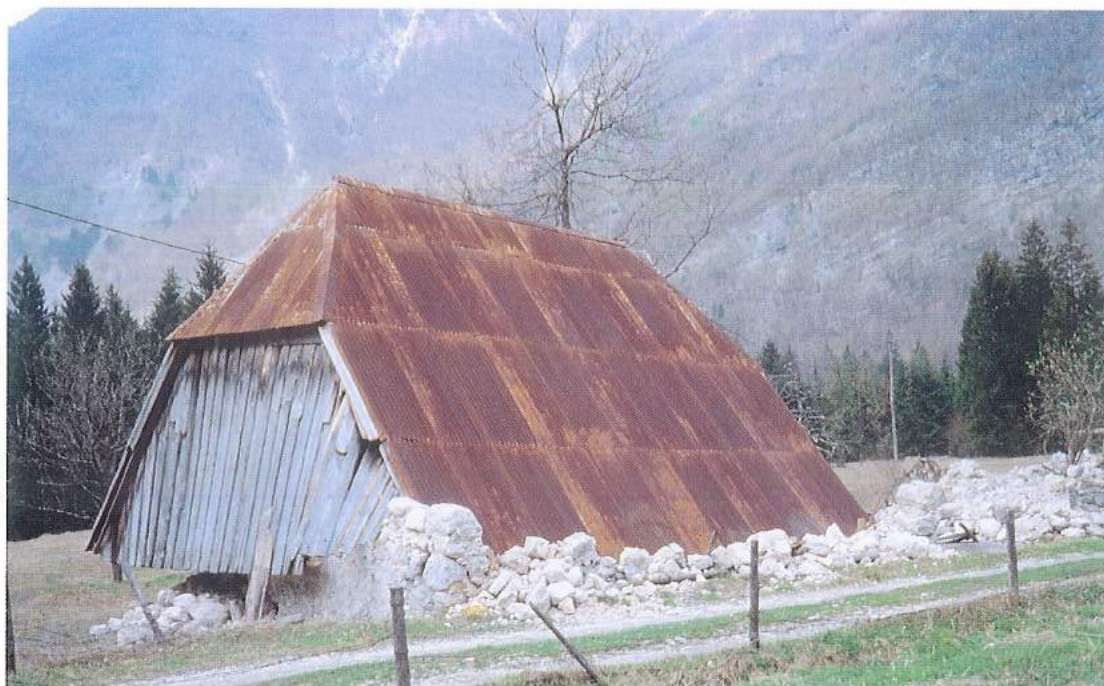
Slika 13. Piš je dosegel tudi nekatere zgradbe. Na slikah vidimo, kako je potresni sunek dvignil lopo, ki jo je kasnejši piš dobesedno premaknil za več metrov. Figure 13. Air shocks also reached some buildings. The figures show how the earthquake shock raised a shed, which the subsequent air shock literally moved on several metres further.
