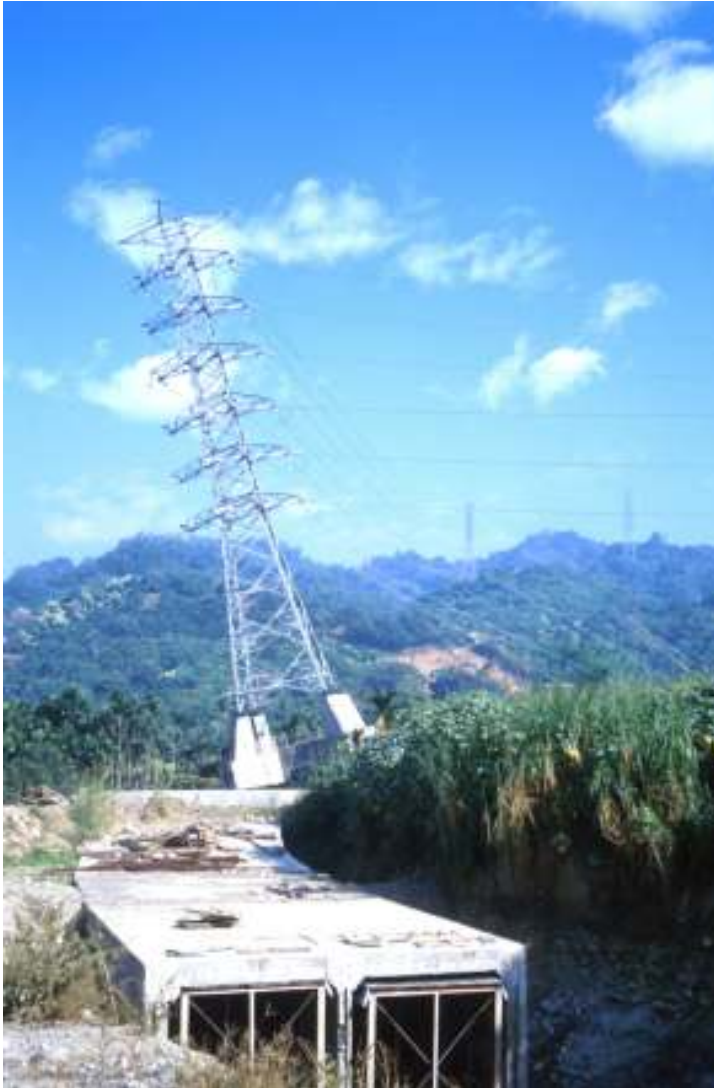
Slika 6. Posledice potresa so bile tudi na daljnovidih. Nagnjenje stebra je posledica lokalnih geoloških pogojev (foto: R. Vidrih). Figure 6. The earthquake also damaged the power supply network. The leaning of the column is the consequence of the local geological conditions (photo: R. Vidrih).
