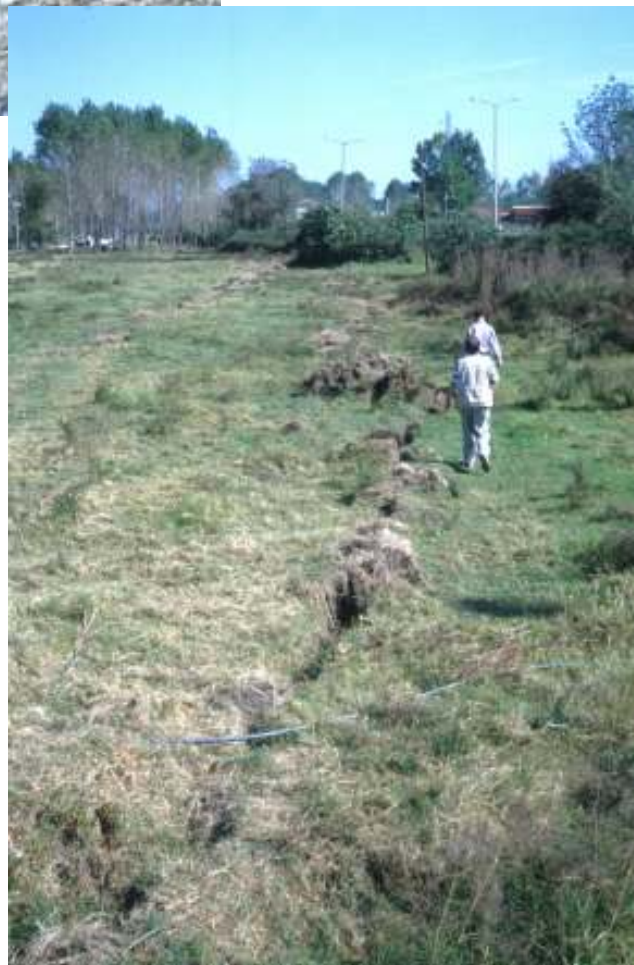
Slika 21. Površinski pretrg ob prelomu je nastal v dolžini 10 km. Vertikalni zamik je bil okoli 60 cm (foto: R. Vidrih). Figure 21. A surface fault rupture along the fault appeared in the length of around 10 km. There was a vertical offset of around 60 cm (photo: R. Vidrih).
