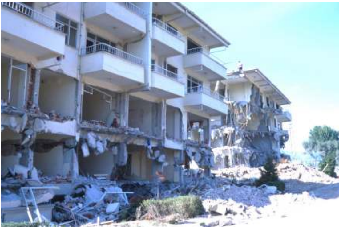
Slika 15. Posedanje objektov zaradi slabih geoloških razmer (foto: R. Vidrih). Figure 15. Subsidence of buildings due to unfavourable geological conditions (photo: R. Vidrih).
