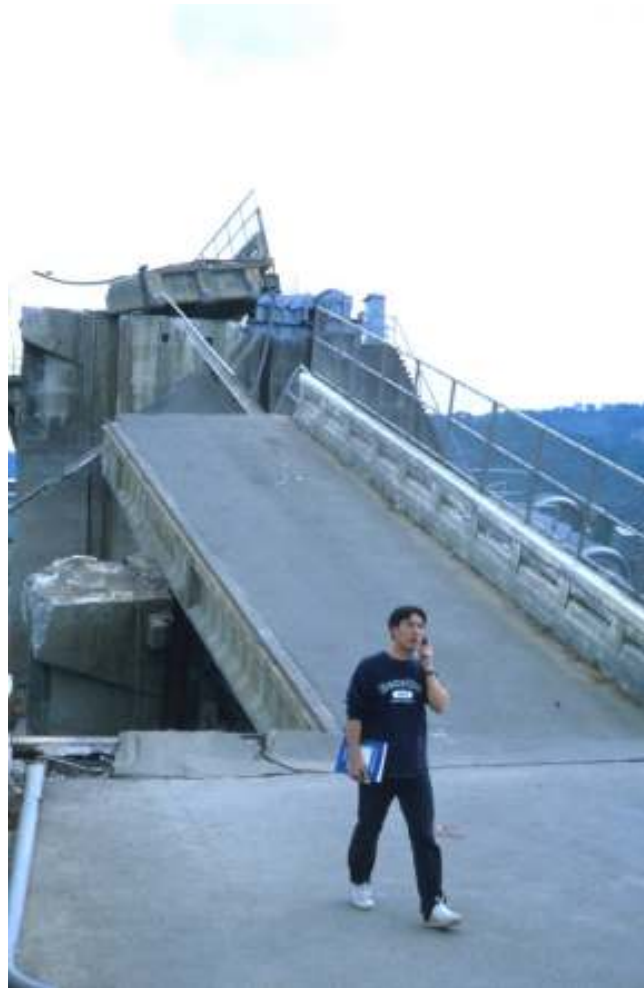
Slika 11. Pred potresom je dovozna cesta čez pregrado potekala vodoravno (foto: R. Vidrih). Figure 11. Prior to the earthquake, the road over the barrier was horizontal (photo: R. Vidrih).
