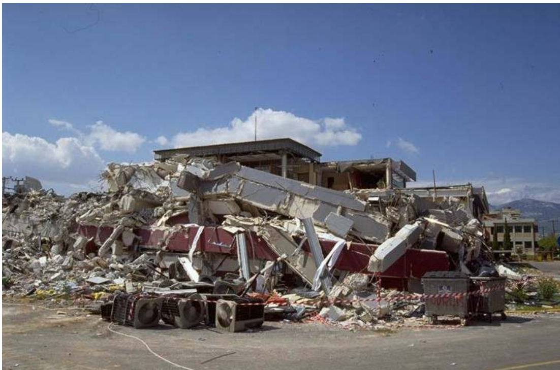
Slika 5. V večjem delu tovarne »Fourlies« so bile težko poškodovane konstrukcije. Figure 5. The factory »Fourlies«, part of the building collapsed and the rest suffered serious structural damage.
