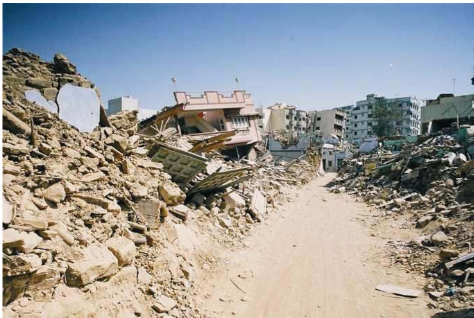
Slika 22. Deli starega obzidanega mestnega središča mesta Bhuj so bili popolnoma opustošeni. Slika prikazuje razsežnosti potresa – veliki predeli so bili uničeni do nerazpoznavnosti, ne glede na to, iz kakšnega materiala so bili sezidani objekti (betonski ali kamniti). Najpogosteje so bili objekti v osnovi iz kamna, na katere so kasneje dogradili armirano betonska nadstropja ali težke AB strehe. To je samo pripomoglo k dejstvu, da se preobremenjena spodnja nadstropja sesedla zaradi teže in togosti zgornjih nadstropij. Figure 22. Sections within the old walled city of Bhuj were completely devastated. This image gives an idea of the extent of the damage – most structures over a many block area were rendered unrecognizable regardless of whether they were reinforced concrete, or constructed of stone. Most often, the buildings were made of stone originally, and later had heavy concrete roofs or top storeys added – which only served to help the overloaded stone structures beneath collapse from the weight and stiffness of the overburden.
