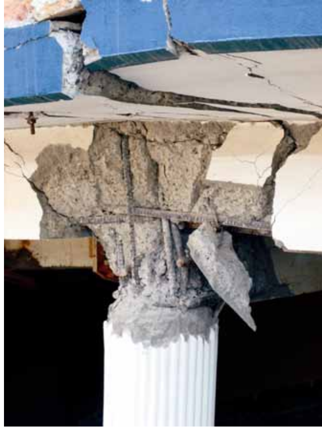
Figure 15. Abbotabad: details of damage of a collapsed r.c. structure - inadequate joint reinforcement.
