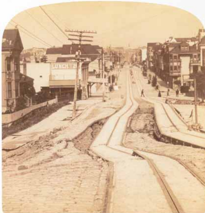
Slika 2. Premiki ob potresu v San Franciscu so ponekod dosegli več metrov. Figure 2. The movements reached a few meters in some places.
