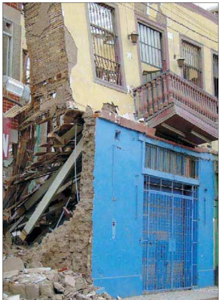
Figures 9a,b. The building made of poor materials and without joins of construction knocked down.
