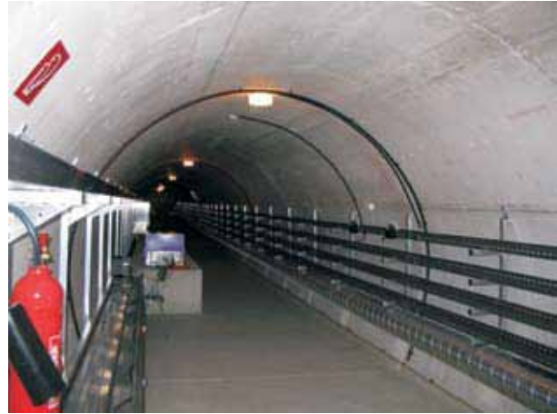
Slika 9. Opravljanje meritev v predoru. Figure 9. Measurements performing in tunnel.
