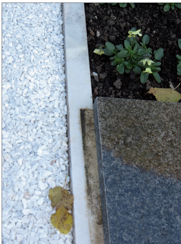
Figure 14: Displaced gravestone at the cemetery in Bušeča vas (Photo M. Godec).
