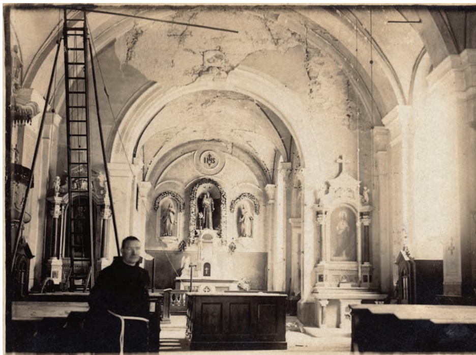
Slika 1: Poškodovana notranjost frančiškanske cerkve sv. Antona Padovanskega v Brežicah (sliko hrani PMB). Figure 1: Damaged interior of the church of St Anthony of Padua in Brežice (courtesy of PMB).
