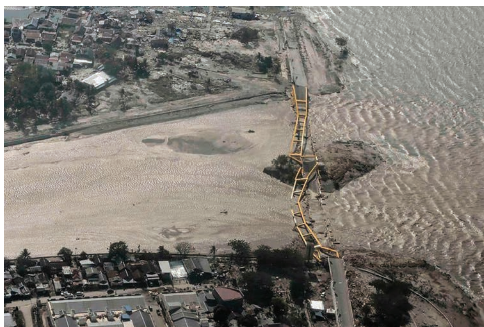
Slika 5: Porušen most Kuning Ponulele (vir: https://www.reuters.com/news/picture/earthquake-and-tsunami-devastate-indones-idUSRTS23EU8 )
